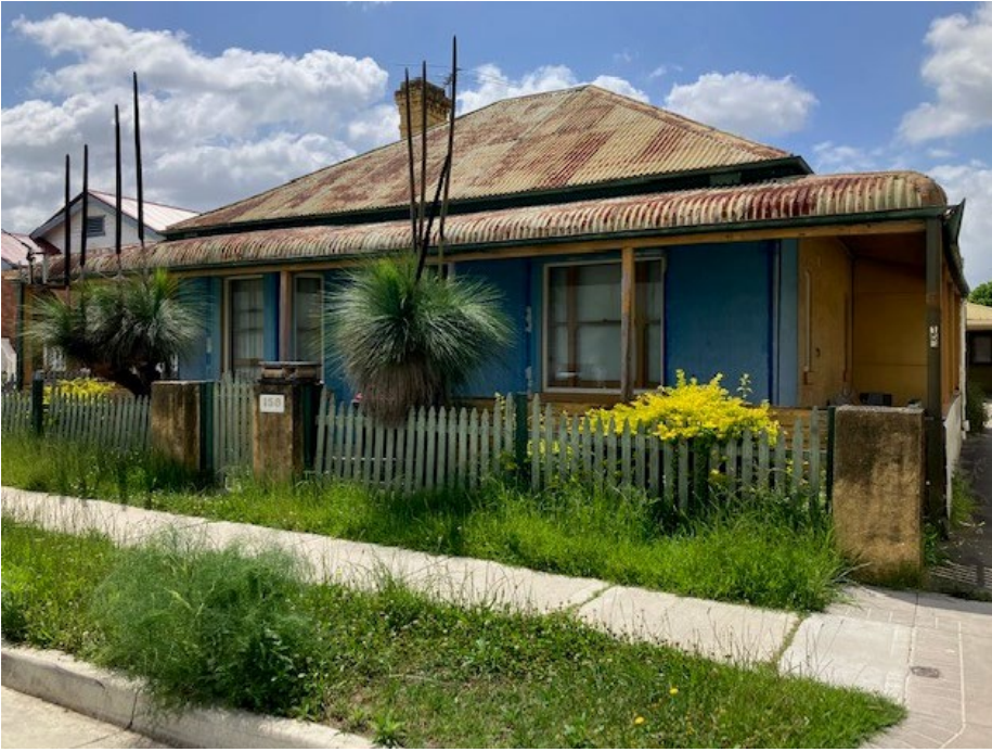
Figure 3: Front elevation of the subject site at 158 Broomfield Street with dwelling house (source: Draft Heritage Assessment, May 2025)
